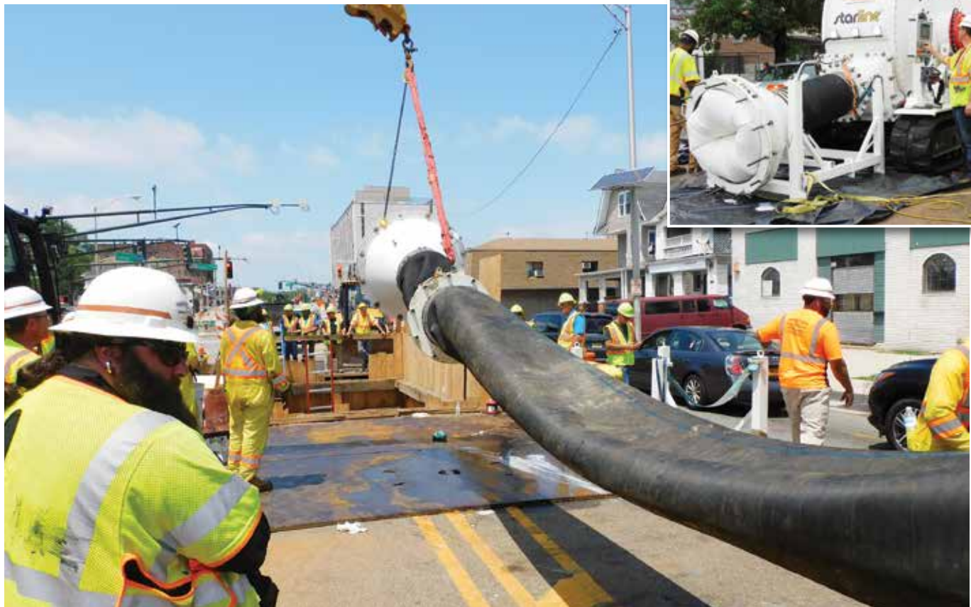
New custom built inversion drum has transport hose for liner
