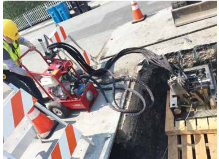
The hydraulically powered extraction machine generates up to 13.3 tons of pulling force and is operated from outside the machine pit
