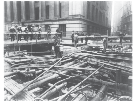
Example of ground congestion at the corner of Wall Street and William Street, Manhattan 1917
