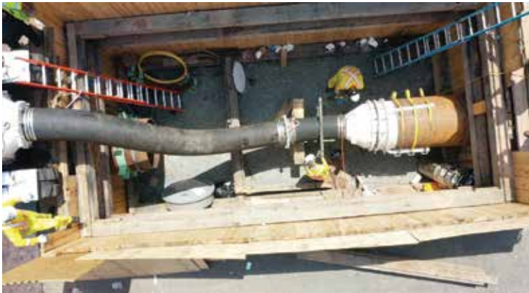
Sending pit, Central Avenue East
