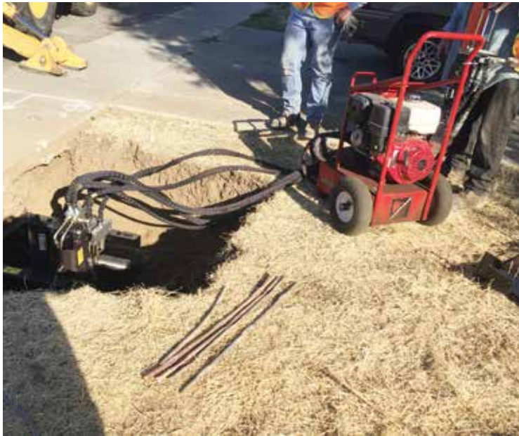
The SLX1300 features onboard pipe shears allowing extracted material to be cut into manageable segments for easy disposal
