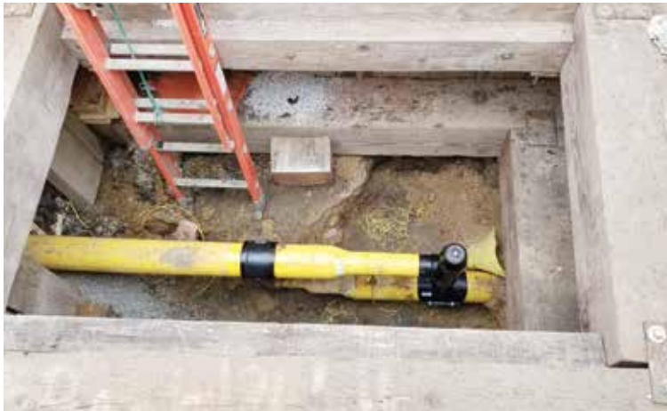
Figure 8 – Site 2: Main Extension for New Service
