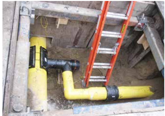
Figure 2 - Supraflow Excavation Pit
