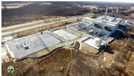
CPV Valley Energy Center Wawayanda, NY 680 MWs Online Fall 2018
